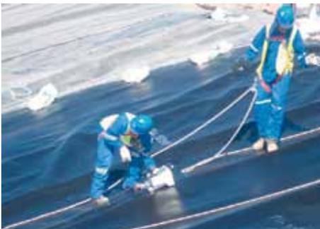
Even uphill to the extreme, the HSK wedge welder HWW 1000 does not face any problems and keeps a consistent speed of movement. Forward movement and optimum heating wedge temperature will be kept, no matter what slope the device rolls up.
