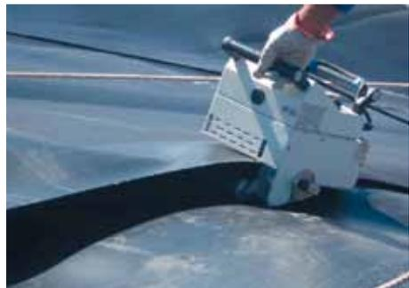
A HSK wedge welder HWW 1000 joints a 2.5 mm PE-HD surface lining.
